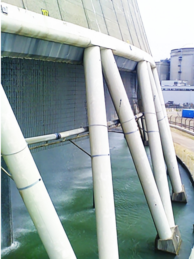
Caption 7: External view of fill packing (counterflow water/air)
