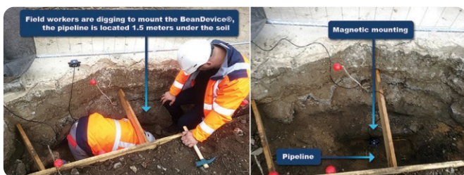
Caption 4: IIOT Vibration sensor installation on pipeline ( BeanDevice® Wilow® AX-3D )
