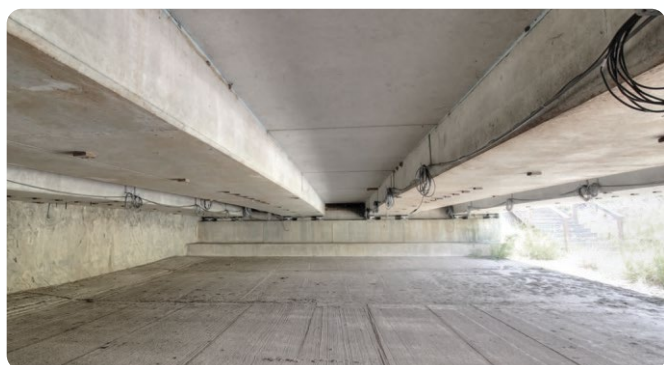
Caption 6: Riverside Bridge – View of the Slab Beams with Cables used for Instrumentation
