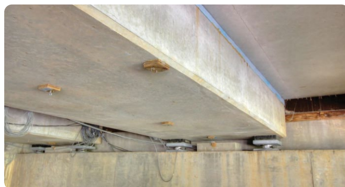
Caption 7: Riverside Bridge – View of the Bearing Pads
